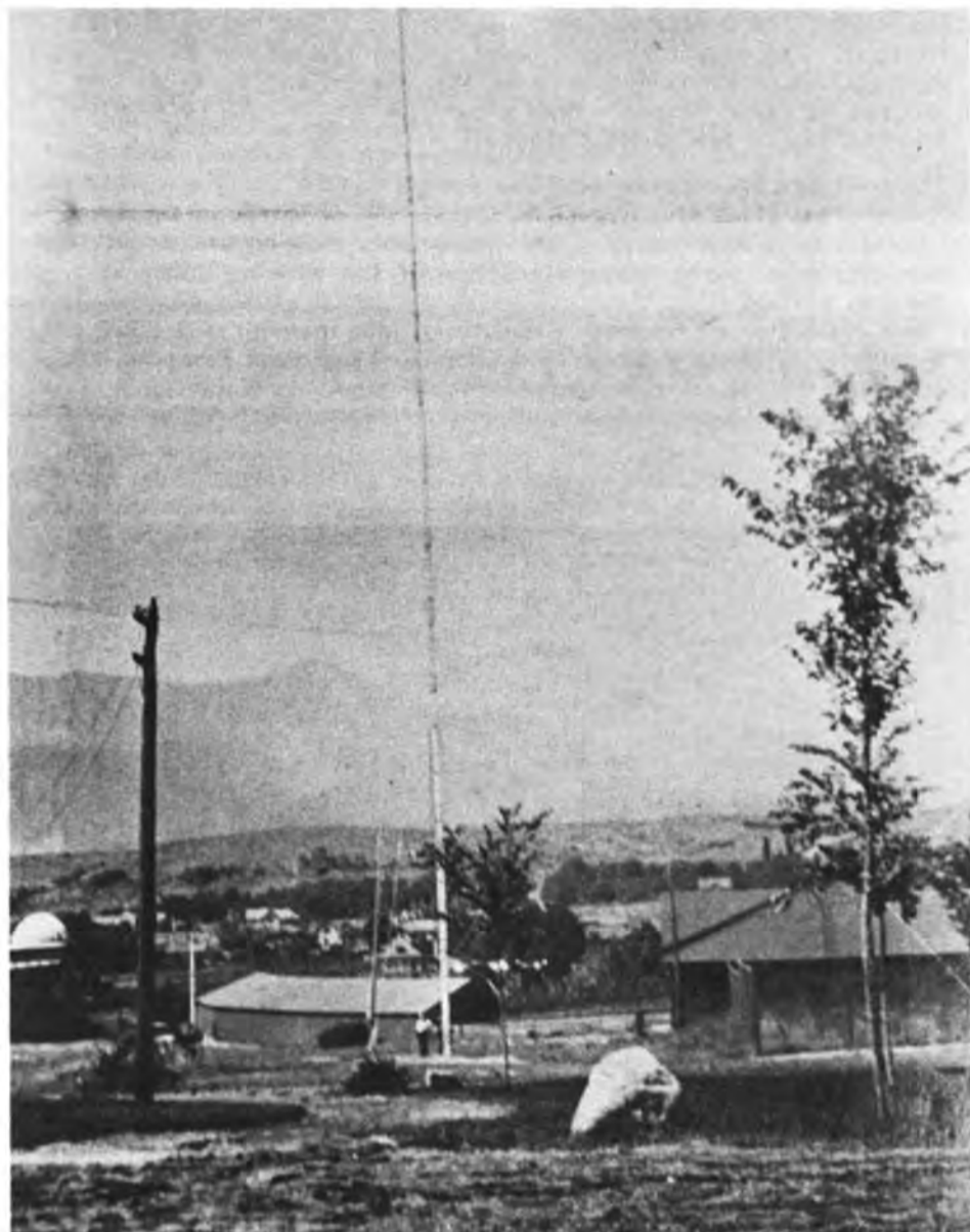
American DeForest Wireless Telegraph Co. radiotelegraph station on the campus of Colorado College, Colorado Springs, CO, June 29, 1905 to Sept. 17, 1907. Call letters "CS". Installed by Charles B. Cooper and Elmo N. Pickerill. Operated and managed by Pickerill. Transmitter: a 2 K.W. open-core transformer, 18-jar Leyden condenser, a spark gap, and a change-over switch. Receiver: electrolytic detector, a three-coil tuner with five slides, and a pair of headphones. The mast is 160 feet high. One of a chain of ten inter-city wireless telegraph stations,---Denver, Boulder, Fort Collins, Cripple Creek, Altman, Pueblo, Trinidad, Leadville, Colorado Springs, Col., and Cheyenne, Wyo.
